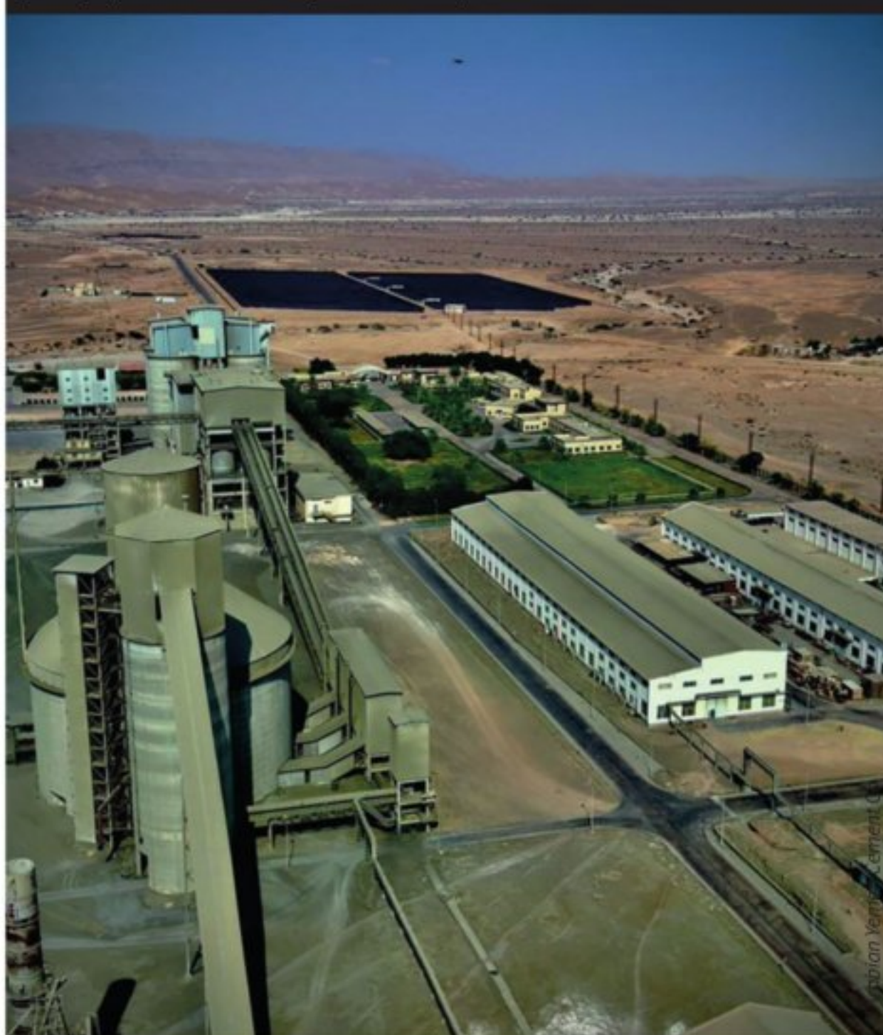
Leading the shift towards renewable energy use in Yemen: Arabian Yemen Cement Co's solar power project at its Hadramout plant in Mukalla, Yemen
