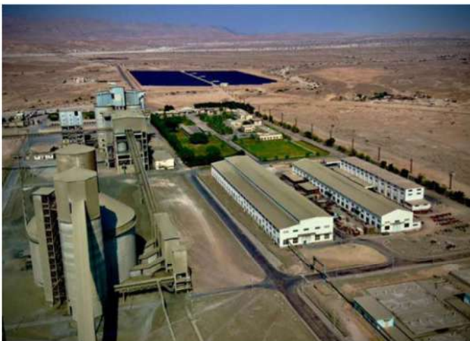
Hydramout Cement Solar Power Plant 13.75 MW.
